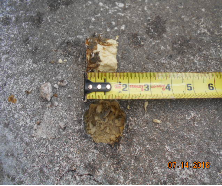
4. ROOF CORE ON AREA "H"
