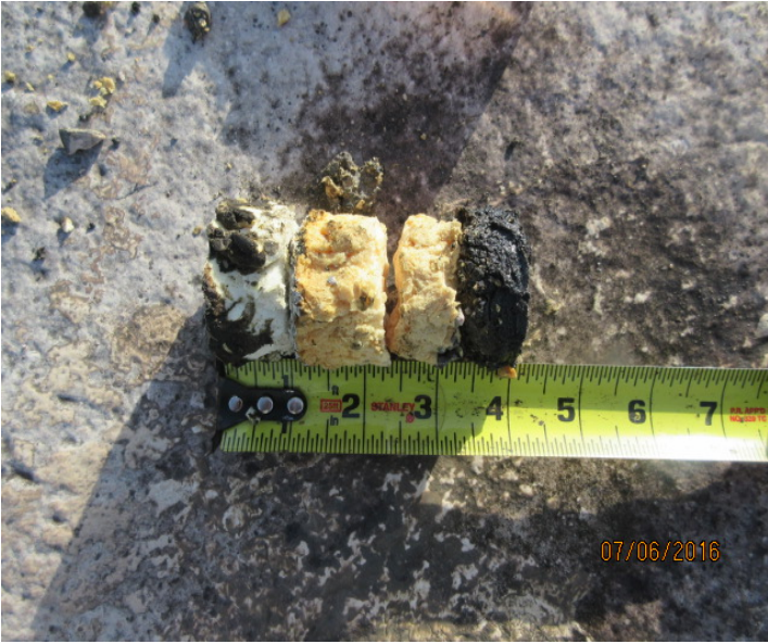
2. ROOF CORE ON AREA "B"
