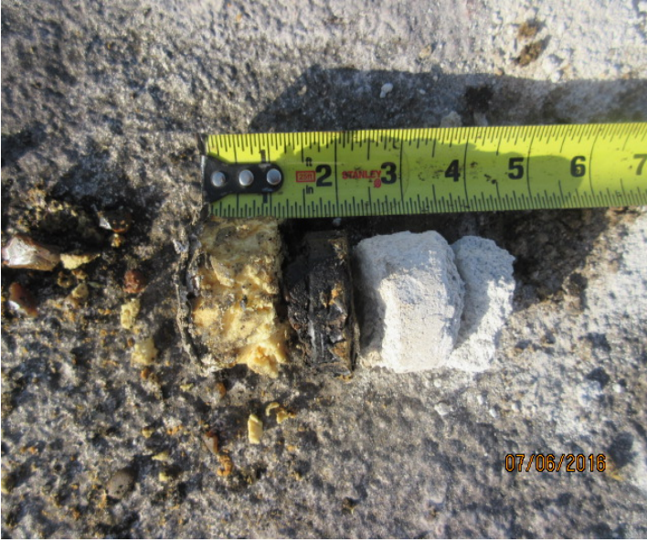
3. ROOF CORE ON AREA "D"
