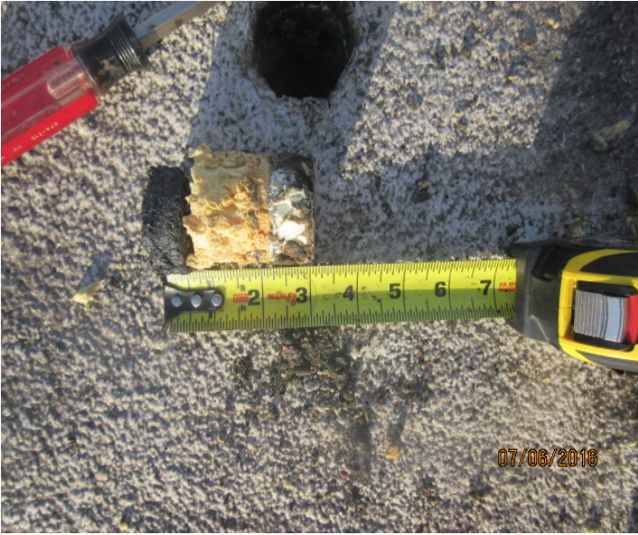
1. ROOF CORE ON AREA "A"
